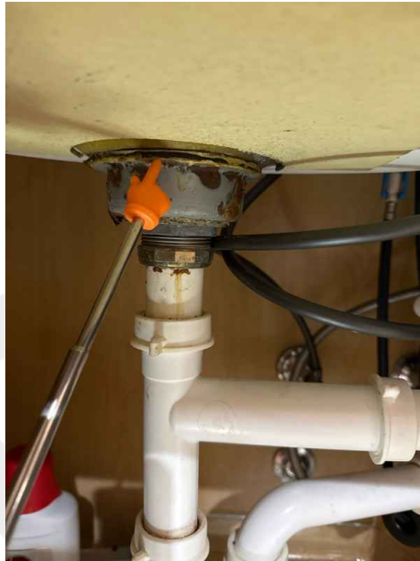
The under sink seal is beginning to a road and shows signs of leaking.
