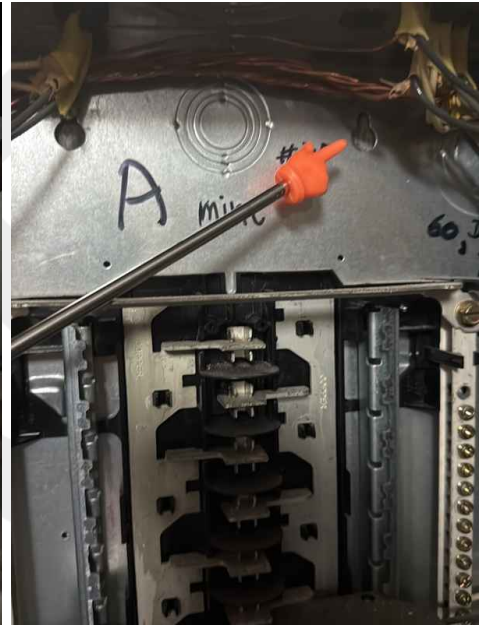
Panel a missing mount screw
