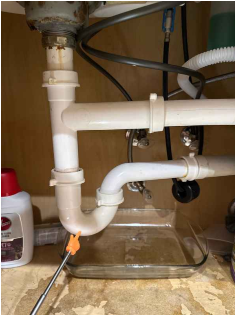
The sink trap should have a drain
