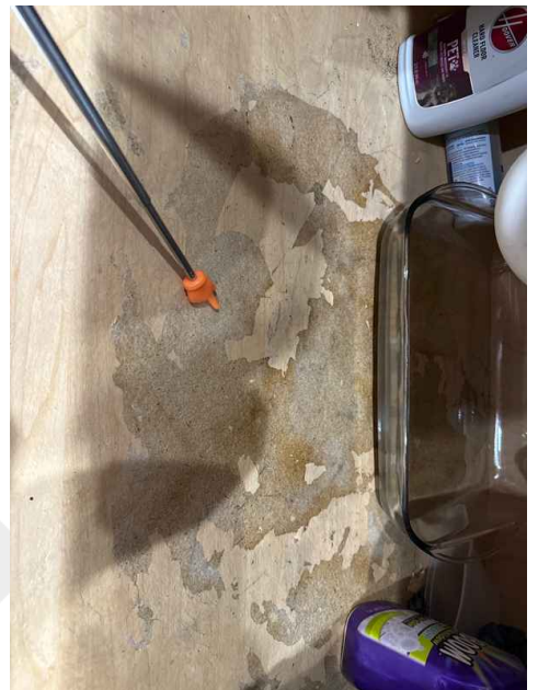
The base of the cabinet looks to have been exposed to significant amounts of water perhaps during maintenance or repair. The area did not show moisture on the meter.
