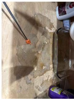
The base of the cabinet looks to have been exposed to significant amounts of water perhaps during maintenance or repair. The area did not show moisture on the meter.
